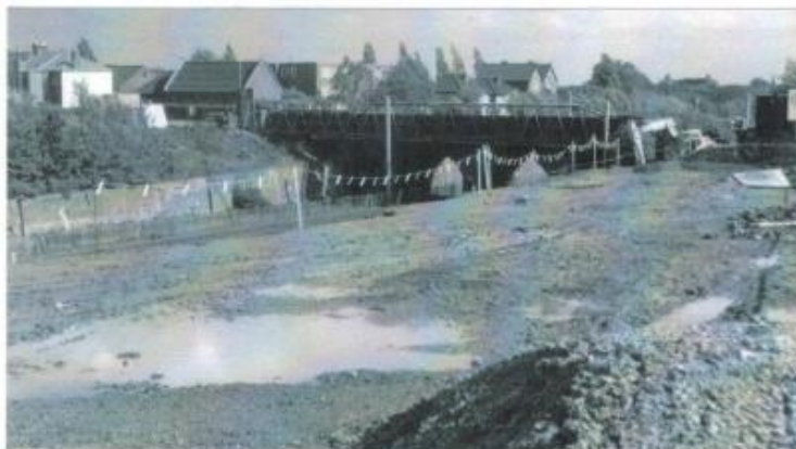
Work starts on the footbridge
