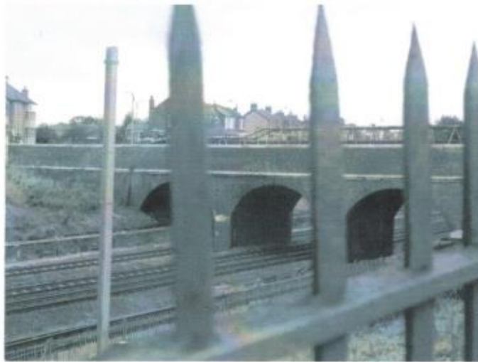
The old road bridge, from the south
