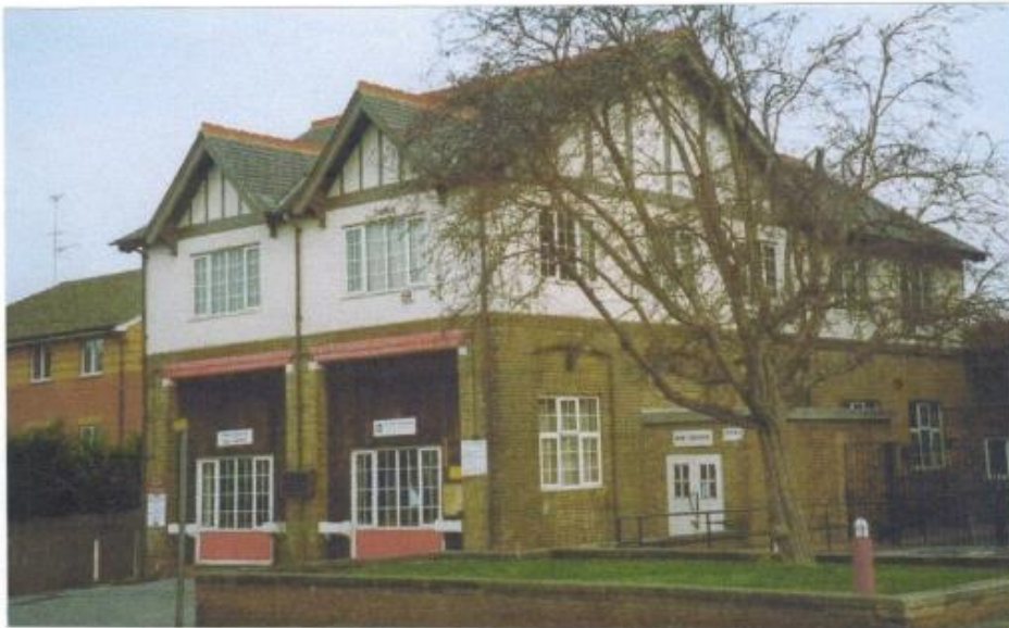
The Day Centre, formerly the Fire Station
