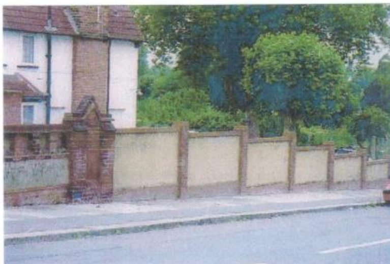
The new wall, with some of the original on the left
