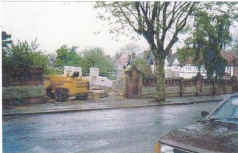
The old wall, with part being demolished, and the tree
