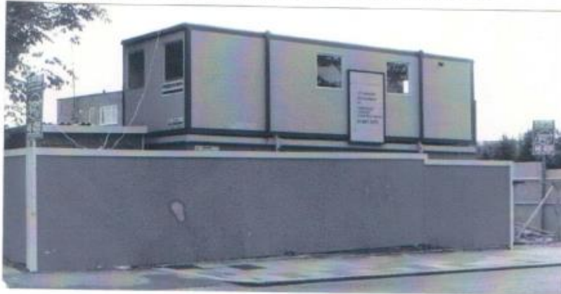
1988. The house has been demolished and builders have moved in
