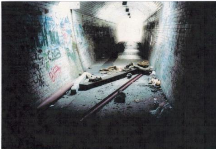
Railway debris, a danger to subway users
