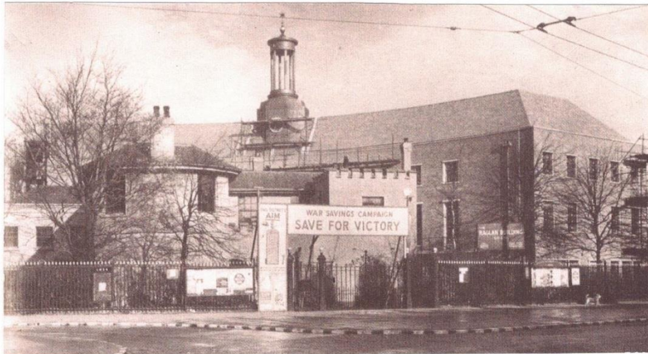
The new town hall takes shape behind The Priory in 1940
