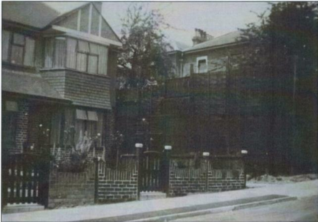
This photograph was taken in 1934 by Friern Barnet Urban District Council as a result of a complaint by the resident of number 4 Cardrew Avenue about the height of the fence adjoining the nudist colony (photo courtesy Barnet Local Studies & Archives)
