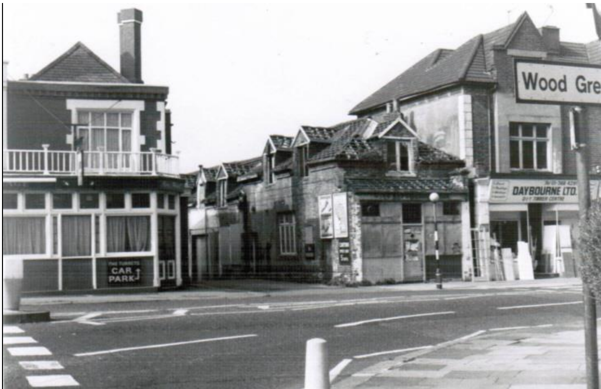
The dilapidated stables, on the right of the picture
