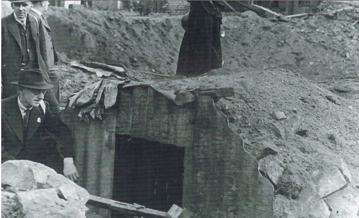
Excavating an Anderson shelter
