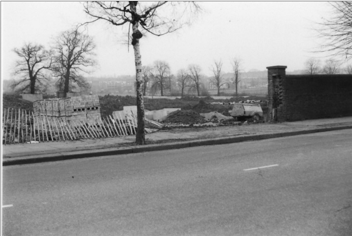
The breach in the wall photographed by John in March 1982. This was to become Firs Avenue.
