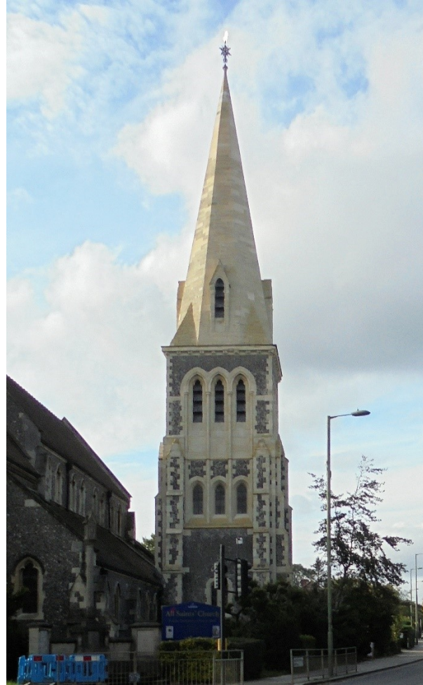
....May 2019 The finished result
